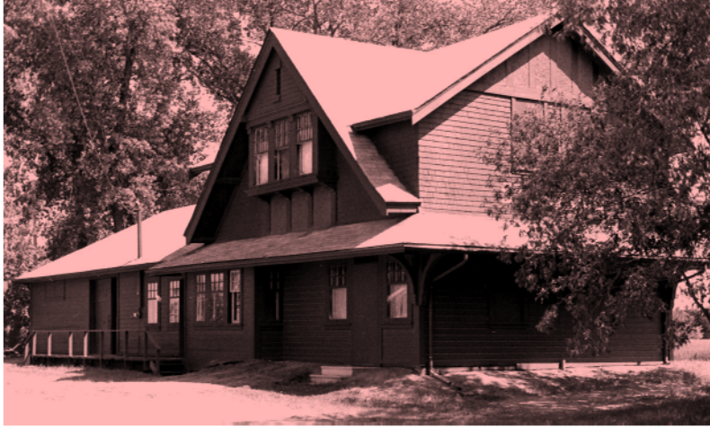
Figure 21 The St. Claude station is a good example of the W.L. "A3" design.
