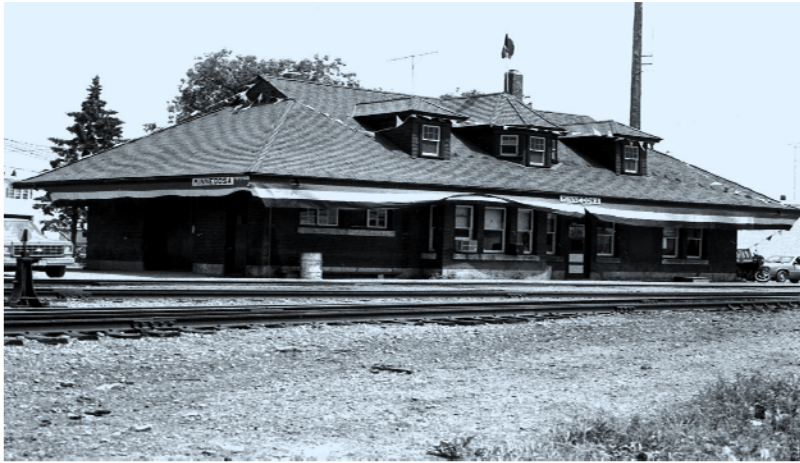
Figure 28 The CPR Station in Minnedosa.
