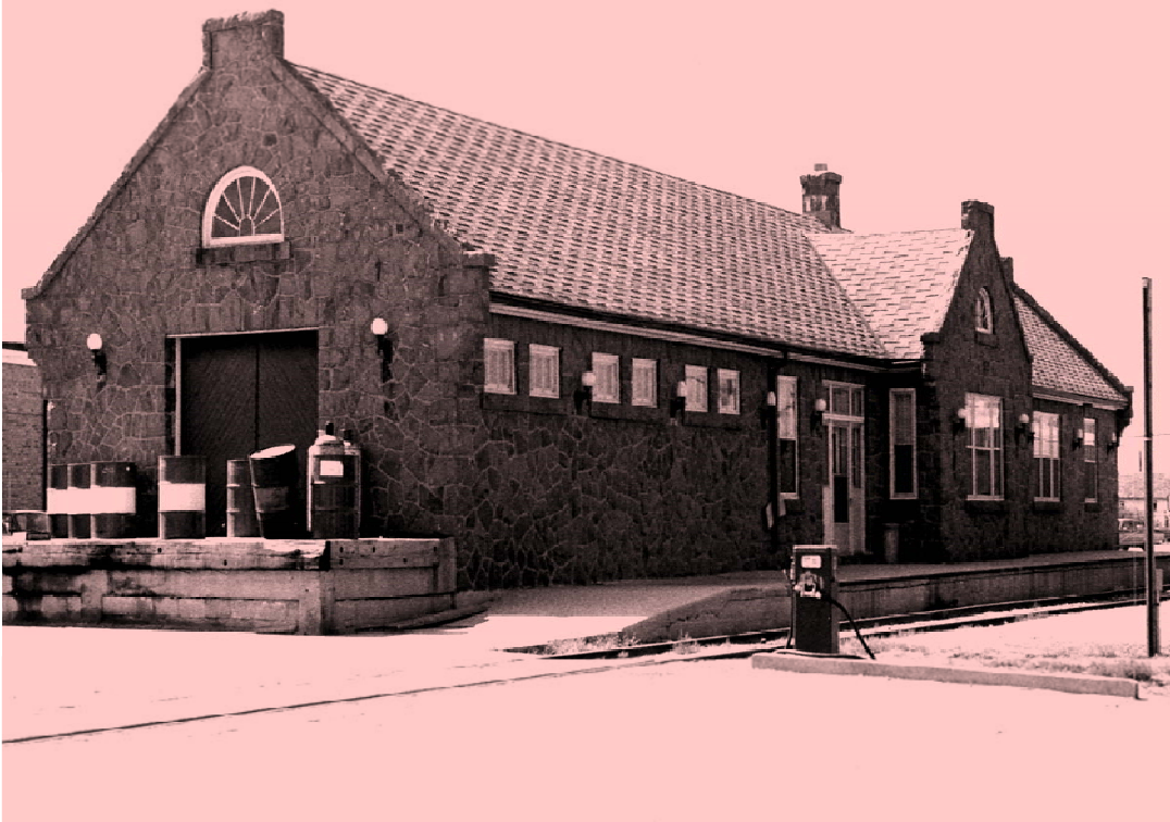
Figure 30 The Greater Winnipeg Water District Station in Saint-Boniface.
